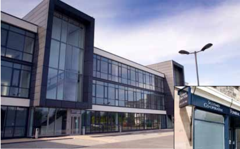
Above: The new office development at Harvest Drive. Right: The new look funeral fascia at Fountainbridge.
